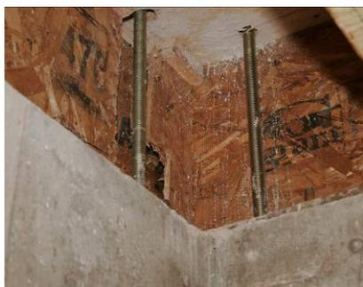
The frame of the home is bolted to the foundation.
