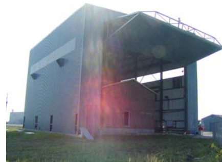
The open door on the steel cover building reveals the full-scale test house within. The structure can be moved by rail to expose the home to the natural elements.
