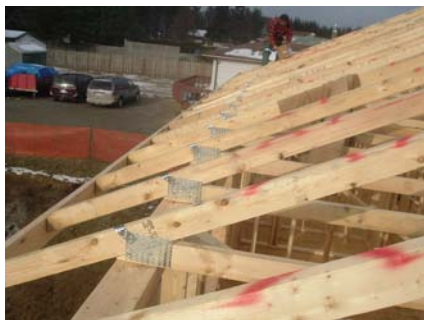
The roof is attached to the frame using special clips.
