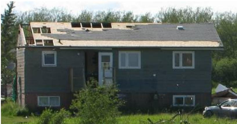
Roof damage as the result of a tornado in Saskatchewan.
