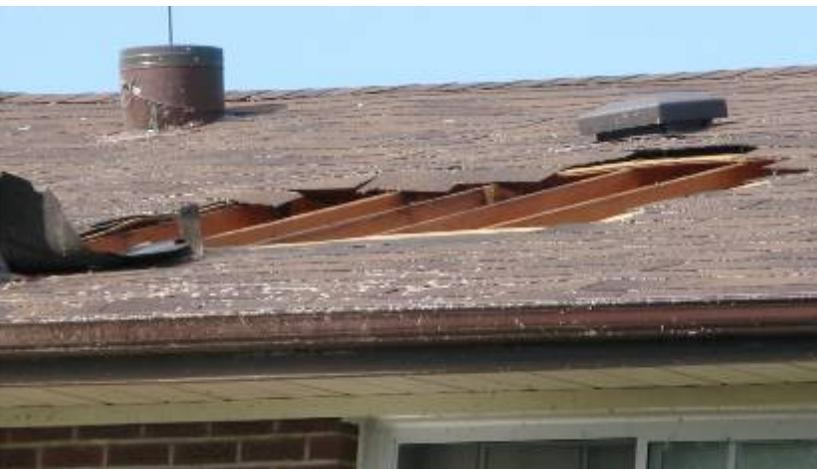
Sheathing failure caused by inadequate hold-down strength, likely missing nails or deteriorated materials, in Vaughan, Ontario.
