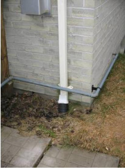
Figure 2: The roof runoff link is directly connected to the storm sewer.
