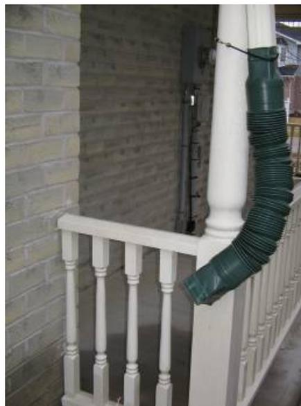
Figure 1: This porch downspout directs water too close to the home's foundation.
