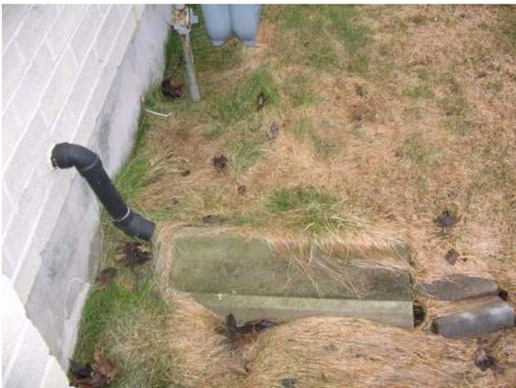
Figure 3: The sump pump discharges too close to the foundation.
