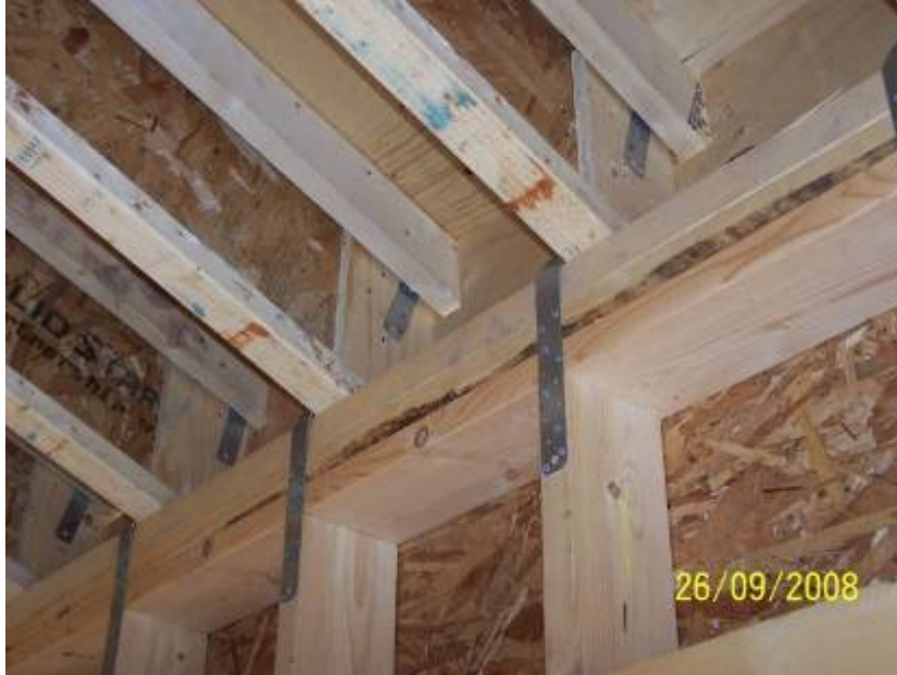
The roof of the home is tied down with hurricane straps.
