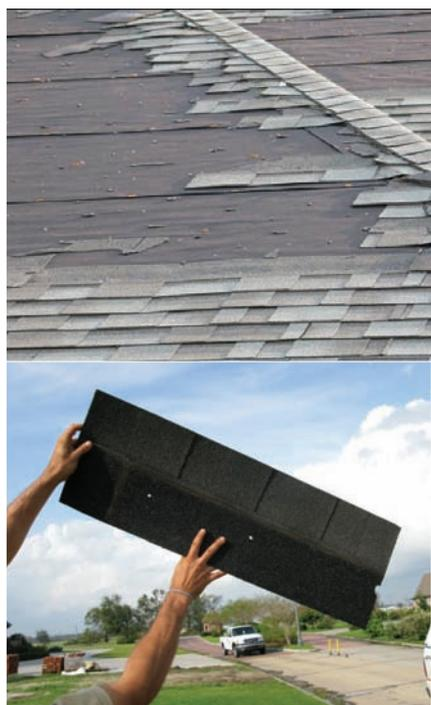
Close-up photographs showing typical shingle failures with the nails still in the roof (left) and one of the shingles that came off with two nail holes visible (right).
