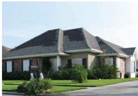
Photograph of a recently-constructed house in Houma, Louisiana the morning after Hurricane Gustav made landfall. The general lack of debris indicates a relatively minor wind event, although one cannot see all of the shingles in the backyard that flew off from the front of the house. Note that this area had been evacuated and no one had yet returned to clean-up; we were the only people here except for Emergency Response Personnel.
