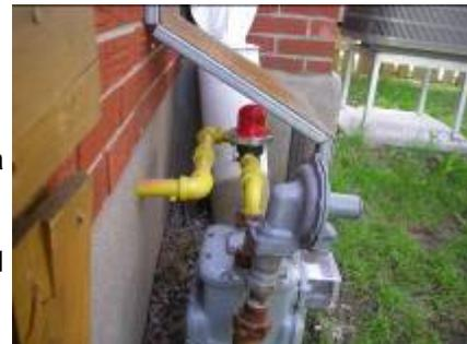
The retrofit included the installation of a natural gas seismic shut off valve and a protective cage, to shield the meter in the event the chimney collapses or other debris falls on it during an earthquake.
