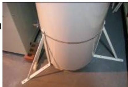
The home’s water heater was fastened to the floor to prevent it from toppling over in the event of an earthquake or other disturbance. This prevents the gas line from severing, causing an explosion and fire, and also prevents water damage.
