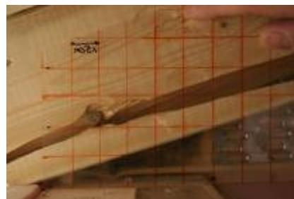
Figure 4: Example of a toenail roof to wall connection in the house where the nail has split the wood and offers very little hold down force.
